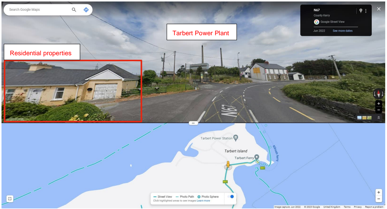
Figure 3-2 View of Tarbert Power Plant from neighbouring residential properties (Google Earth, August 2023)
